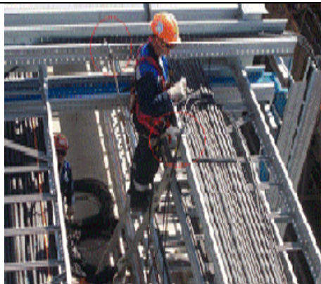
Figure 2: Cable pulling process and posture on tray
